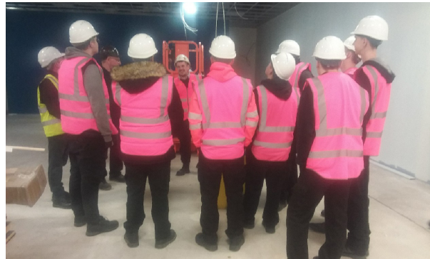
Electrical students site visit (1/2)
